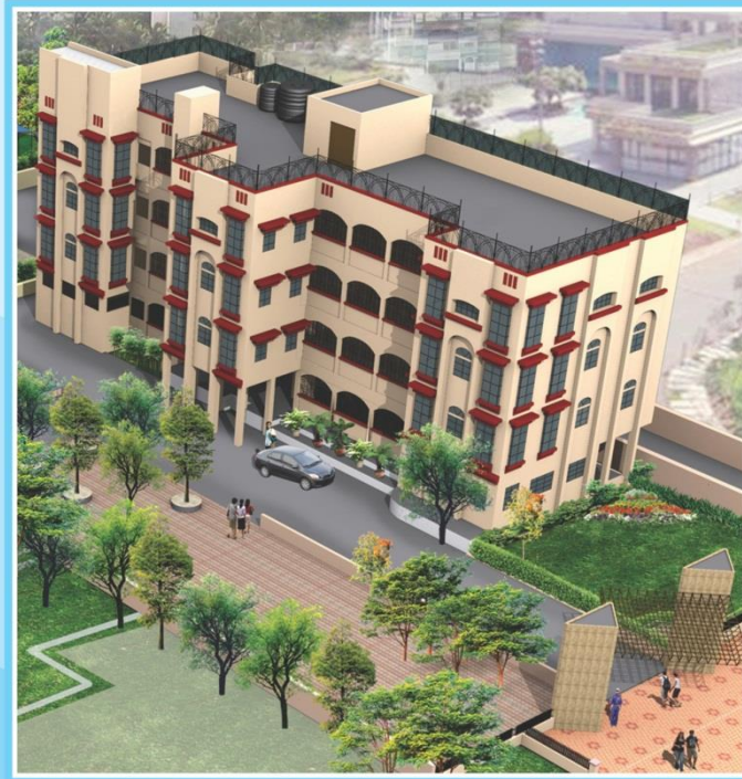
IMS - MAIN BUILDING
